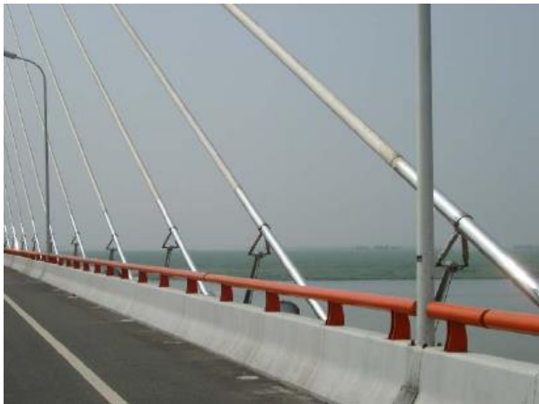
磁流变液阻尼器应用于洞庭湖大桥的斜拉索的风雨振动 Magnetorheological fluid damper used in Dongtinghu Bridge to control the rain-wind induced vibration vibration of the stayed cables
