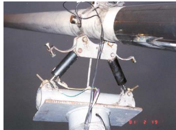
磁流变液阻尼器应用于洞庭湖大桥的斜拉索的风雨振动 Magnetorheological fluid damper used in Dongtinghu Bridge to control the rain-wind induced vibration vibration of the stayed cables
